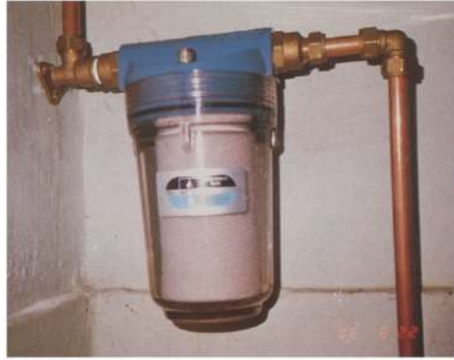
MAIN PIPE INSTALLATION
